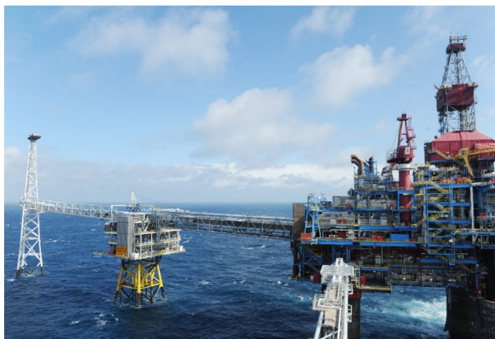
Figure 9. The Sleipner platform with the CO 2 separation unit in the centre (Source: Statoil)
